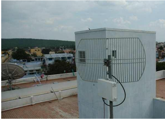
Figure 6: The Theni to Vjerani link in the Aravind network was completely obstructed by a newly constructed elevator shaft. This problem was not resolved until we visited Theni after 2 months.
