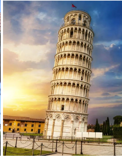
Leaning Tower of Pisa
