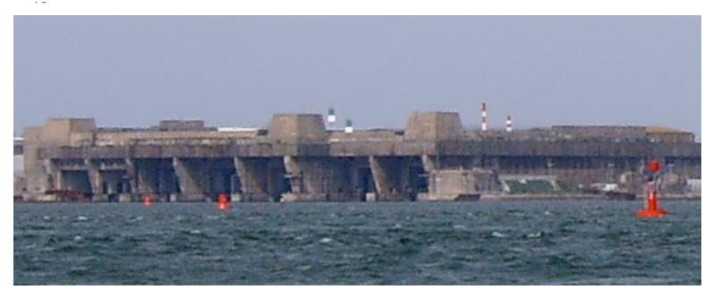
Germans built these U-Boat pens using forced French labor at Lorient on the north coast of the Bay of Biscay. Similar pens were built elsewhere in France, Holland, Norway and Germany. Concrete roofs are several meters thick and surmounted by "Flak Towers" that held 88 mm. guns to discourage aerial attack. Conventional one-ton bombs made little impression on these pens.
